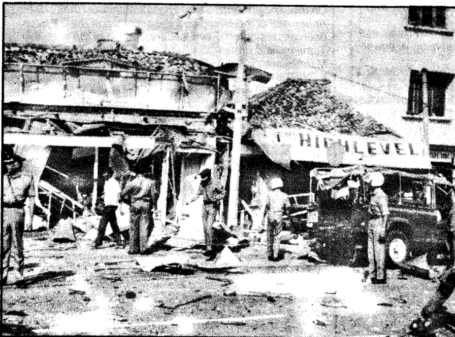
Several buildings in the vicinity were damaged beyond repair
