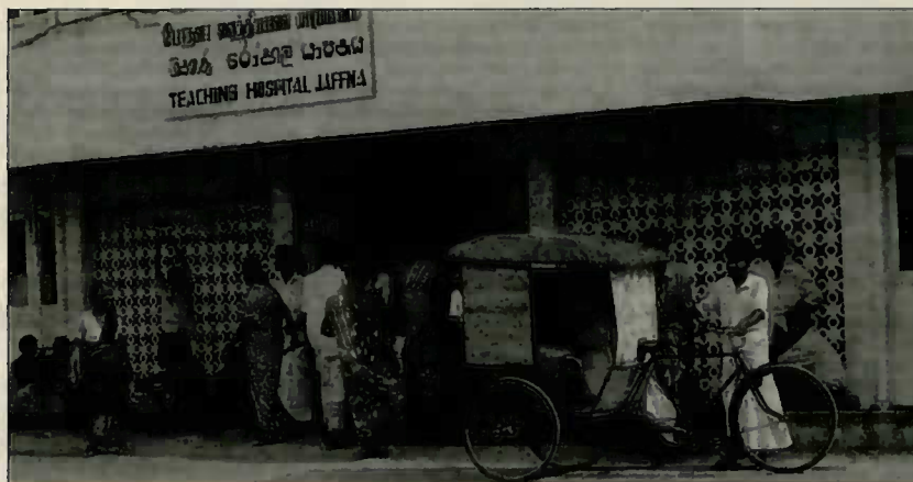
The Jaffna Teaching Hospital: A major portion of the hospital is reserved for the army
