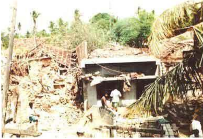
A two story buliding completely collapsed
